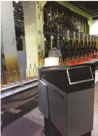
FlexRadar installed on a Bucher Emhart Glass NIS machine.
