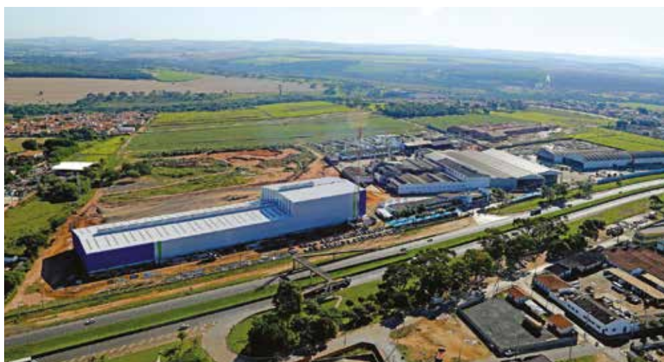
The Vidroporto glass container plant at Porto Ferreira has increased manufacturing capacity to 200,000 tonnes/year.
