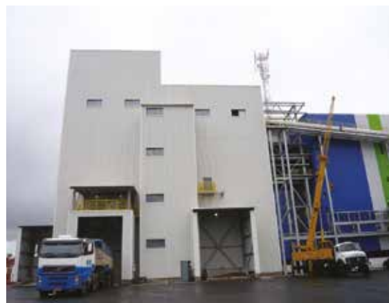
The ZIPPE batch house is designed for the production of 400 tons of batch in 16 hours.
