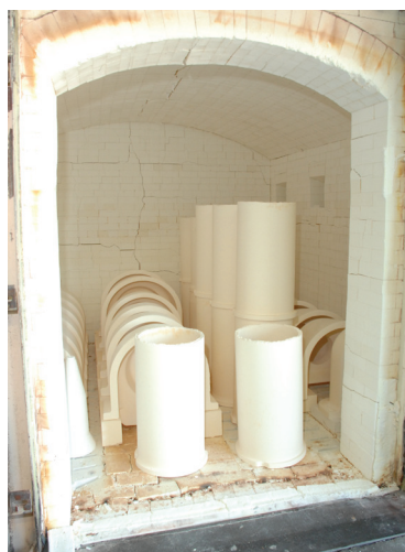
Optimised drying technologies at the Owensville plant.
